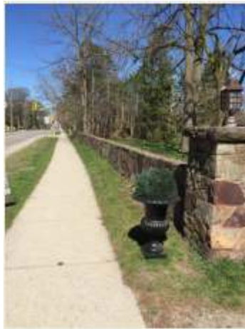
Figure 6.14. Stone Wall in Front of 372 Lakeshore Road West
