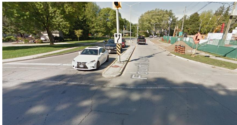
FIGURE 10: Raised Island Protruding in to the North Crosswalk at Fourth Line
